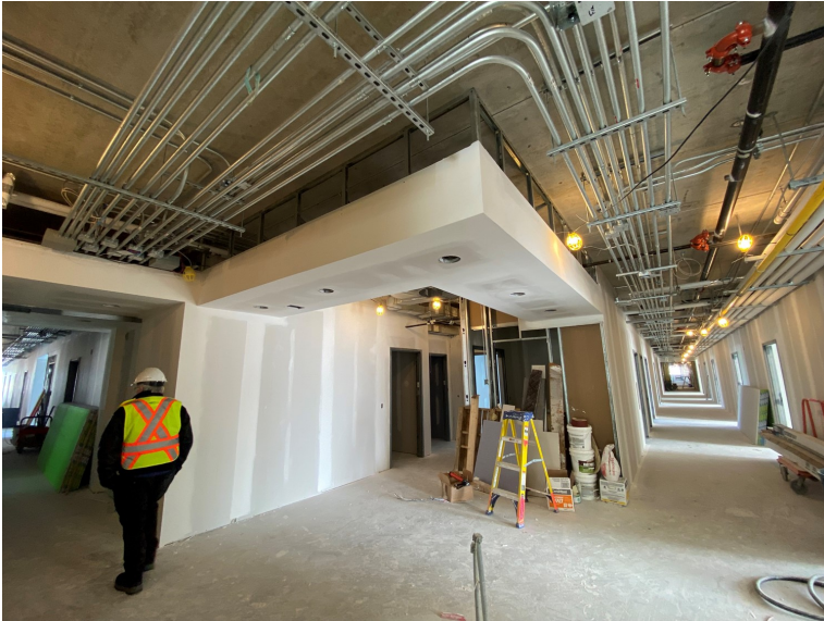
Drywall bulkheads underway.
