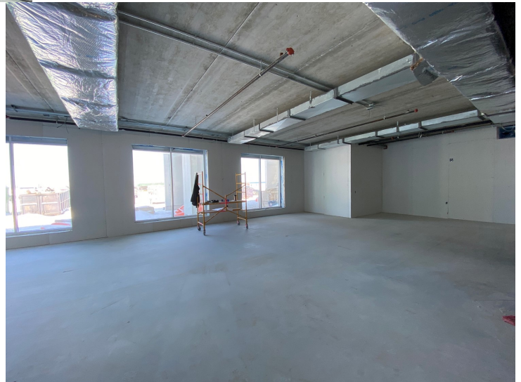
Dining room drywall ready for taping and sanding.
