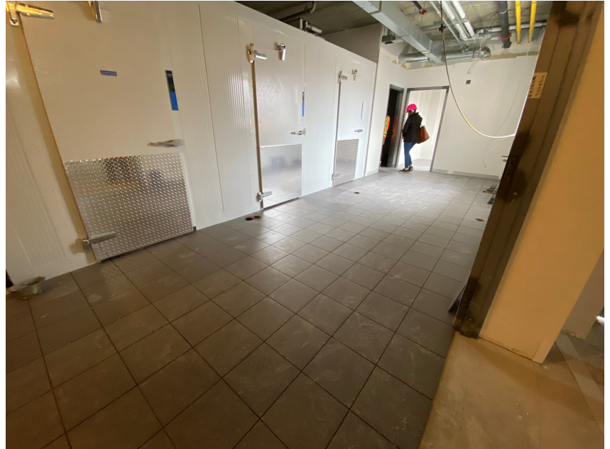
Kitchen fridge and freezers installed. Kitchen tile underway as well.
