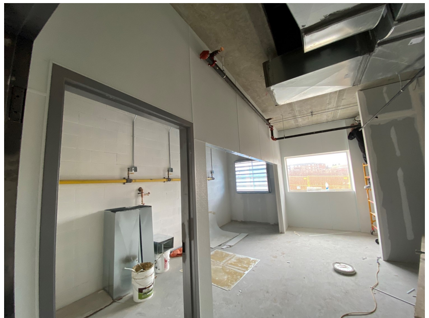
Laundry room hygienic wall paneling underway.
