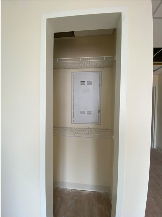
Suite closet shelving and media panels are being installed.
