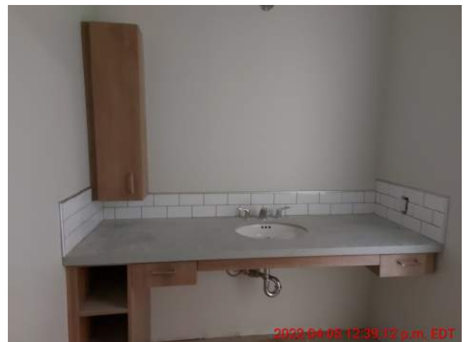
Ensuite vanities underway.
