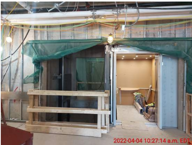
Second elevator cab installation ongoing.
