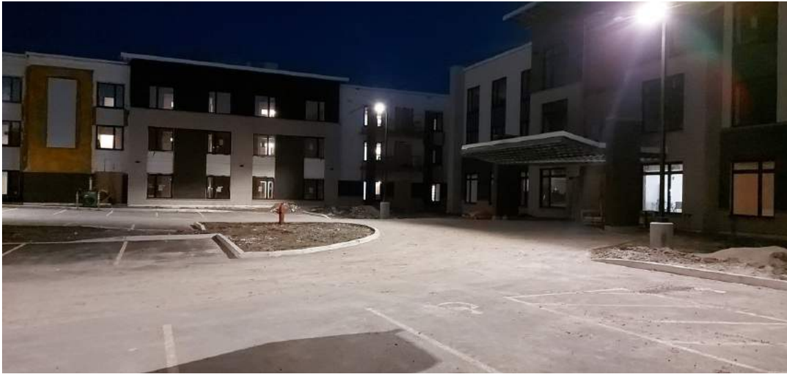
Parking lot light poles installed.
