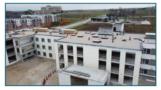
Roof aggregate is in place which helps protect underlying roof layers from UV rays, hail, etc.
