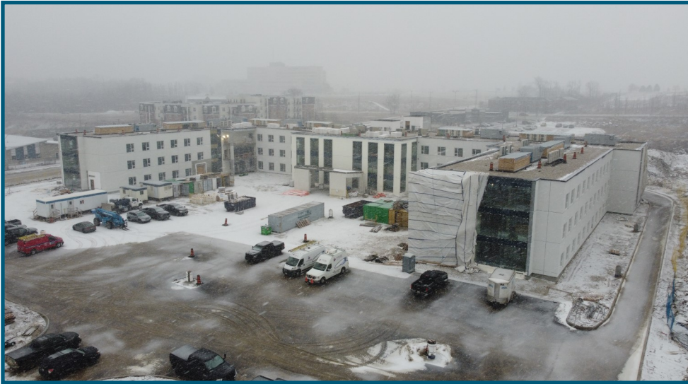
Curtain walls and spandrel panels have been installed.
