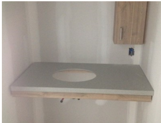
Washroom vanity millwork in mock-up suites underway.
